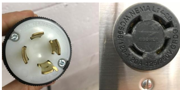
Figure 7: NEMA L14-20 type plug and required outlet.
